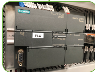
Programmable Logic Controller (PLC) provides flexible operation and overall controlling of machine according to the user needs.
