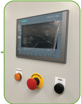
Touch screen control panel with user friendly interface for convenient operation in both automatic and manual function.
