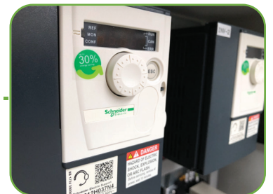
Inverter controller for Screw shafts and Mixing agitator speed adjusting.
